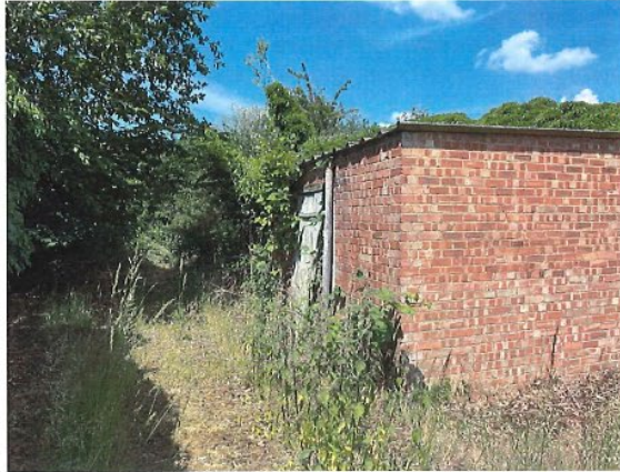
Redundant Farm Buildings
